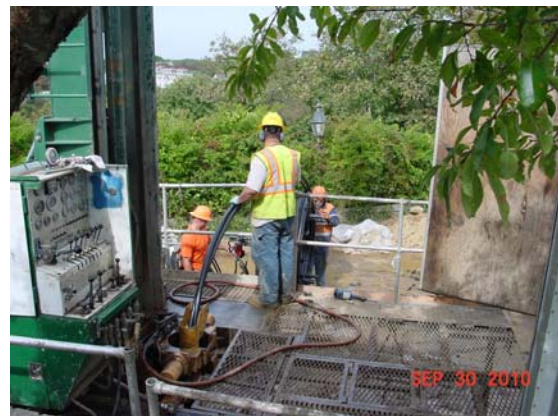
Ground heat exchanger (U-tube) installation in progress.
