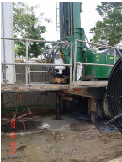
Sonic drilling in progress.
