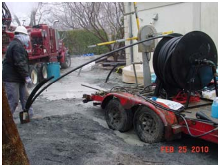
Grouting of boreholes
