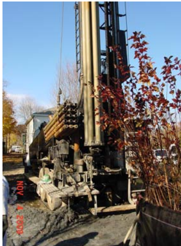
Compressed air rotary DTH hammer drill rig was used to drill the vertical boreholes.
