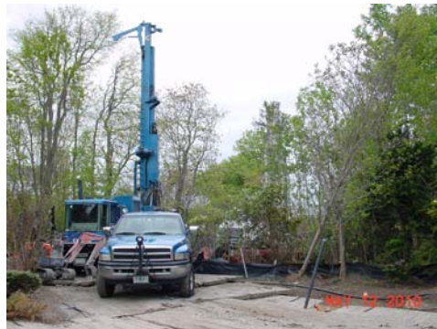
62 vertical boreholes were drilled
