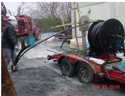
Grouting of boreholes
